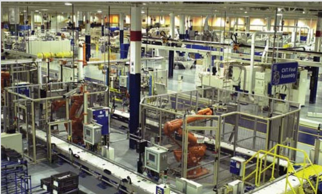
All plant equipment can run on a single network for control and safety
