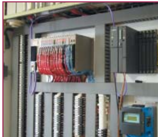
FIG. 4 (left): Holston's PCS 7 system consists of three operator stations in the control room, four operator stations in the production buildings, a S7417 hot backup PLC, three S7416 PLCs, and a 545 PLC. FIG. 5 (right): A redundant H1 network connects a series of redundant PLCs. Profibus is used for control at the cell level.
