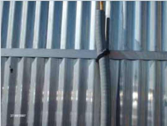
Fig. 11: Conduit open at the top for rain
