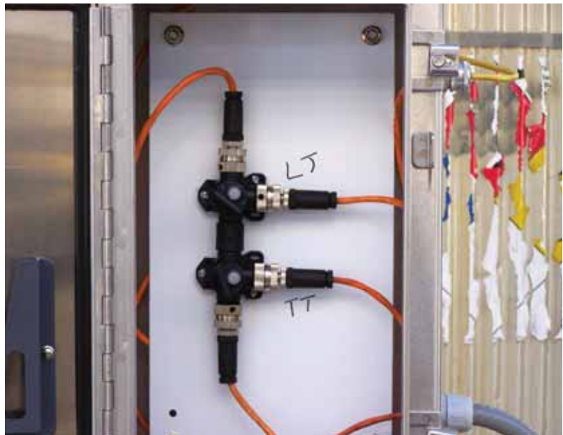
Figure 7: "T" connector junction box with M12 connectors
